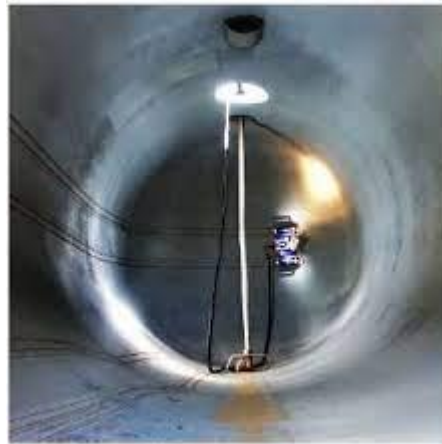
Figure 1 – Magnetic Crawler Conducting Inspections [1]
